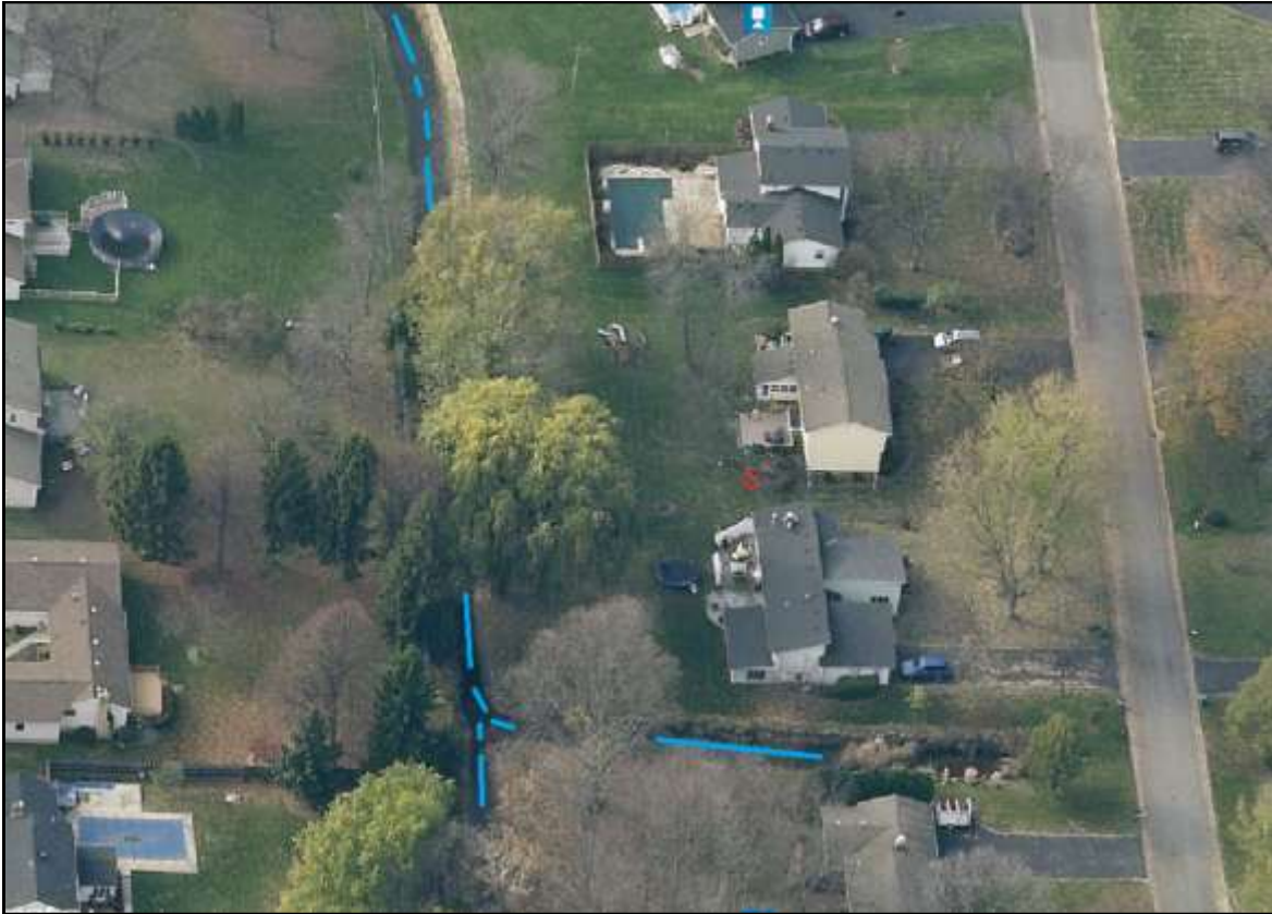
Figure 5. Tufa Glen Creek (blue dashed line) rock-lined and channelized
