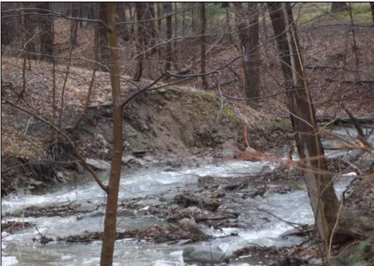
Figure 4. Eroded Streambank downstream of Creek Street on Tufa Glen
