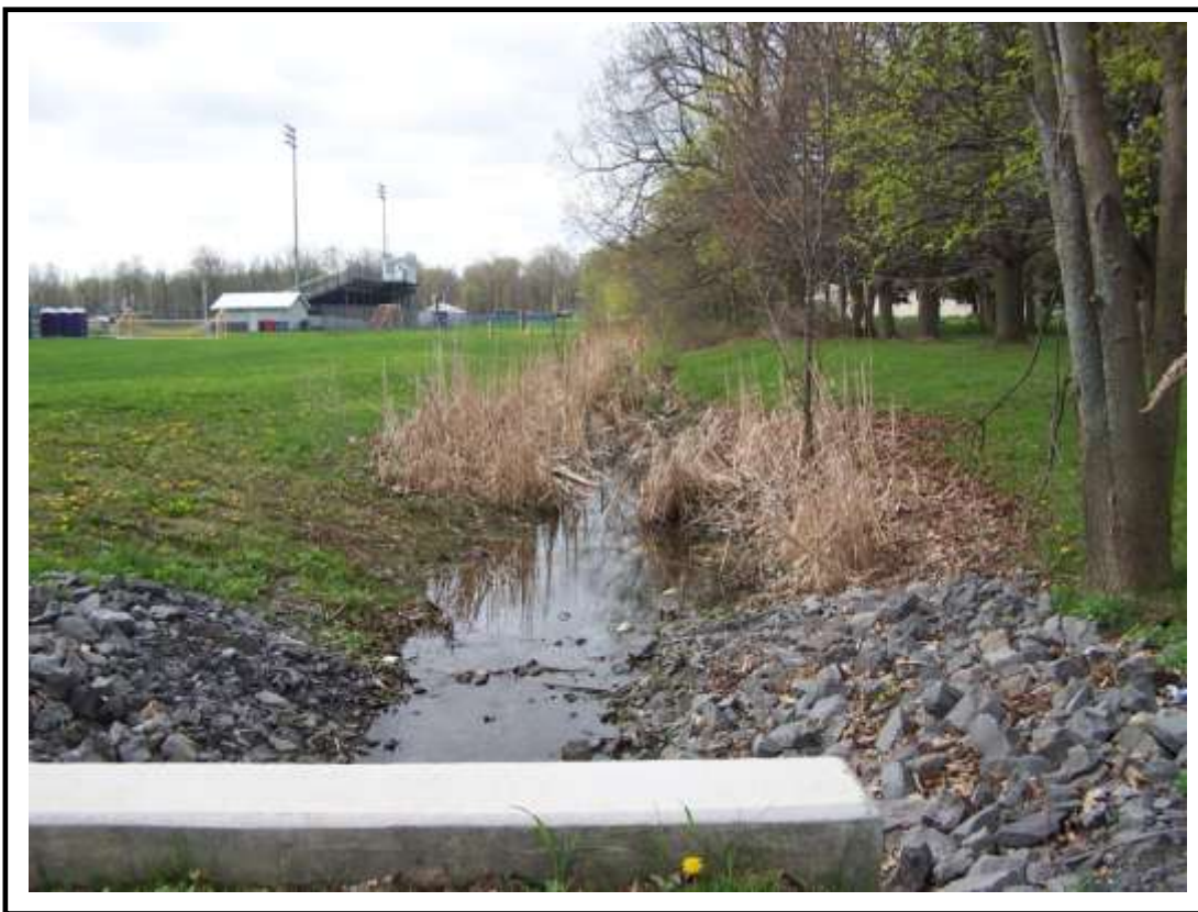
Figure 13. Impacted Buffer at Webster Schroeder High School with High Restoration Potential
